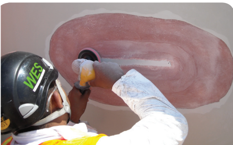
A maintenance technician from Wind Energy Services Company sands the substrate of a blade before applying a surface coat.
