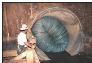
Inserted liner for repair
