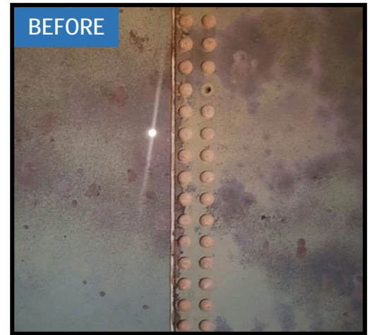
The white spot seen here is daylight showing through holes in the tank.
